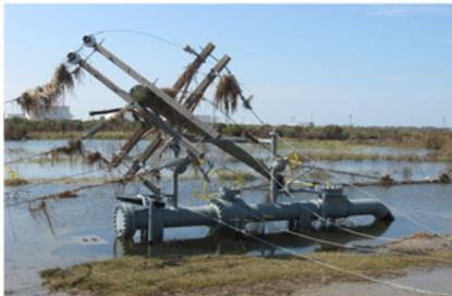
Pipeline manifold impacted by flooding
